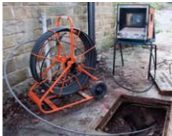
A correct and up to date drainage plan is required by the Control of Pollution (Oil Storage) (England) Regulations 2001 and the Ground Water Regulations (1998) .
